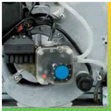
Air pressure switch
