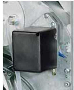
Air-damper opening mechanism
